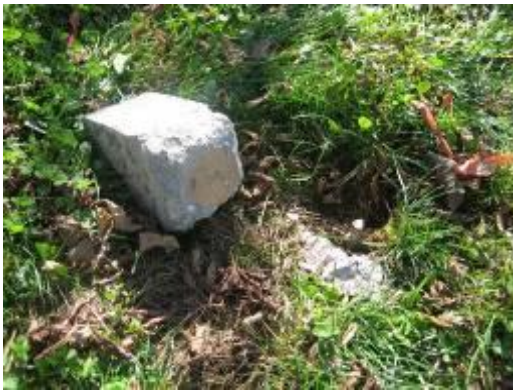
Figure 1. Broken survey monument at the northeast corner between the VYCC and Cowles properties on 10/22/2007. As of 10/21/2009, the monument has not been replaced.
