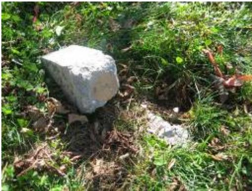
Figure 1. Broken survey monument at the northeast corner between the VYCC and Cowles properties 10/22/2007. As of 11/30/2008, the monument has not been replaced.
