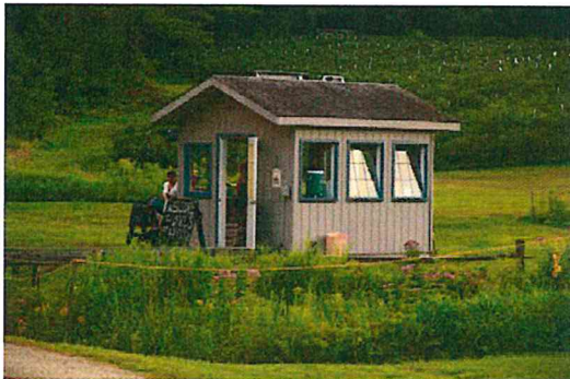
Photo 23: Sales shed, facing SW
