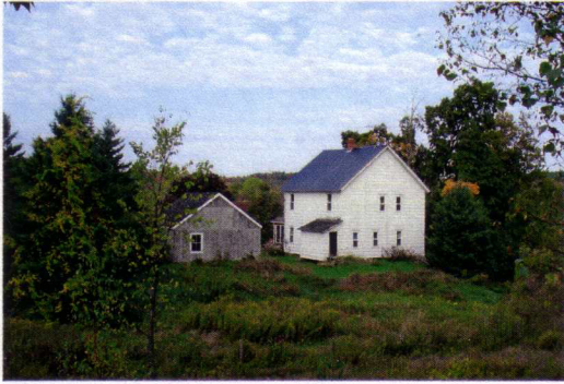
Farm House and Garage
