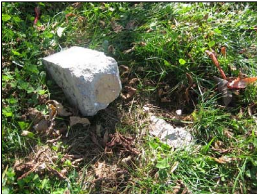
Figure 1. broken survey monument at the northeast corner between the VYCC and Cowles properties 10/22/2007
