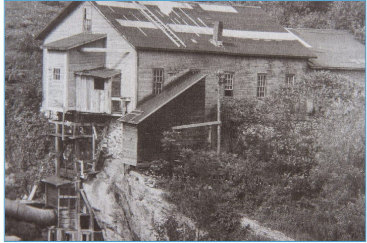
The Richmond Power and Light hydroelectric facility at the Gorge constructed in 1902 provided electricity to the village of Richmond.
